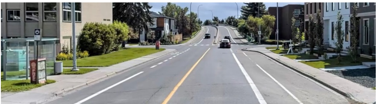
Figure 4.4: Existing Roadway (26 Avenue SW)
