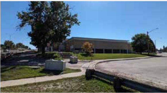
NE Corner of Site
