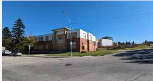
NW Corner of Site
