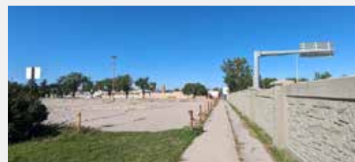
Existing Pathway in ROW East of the Site & Wall Southerly Portion of Site (looking north)
